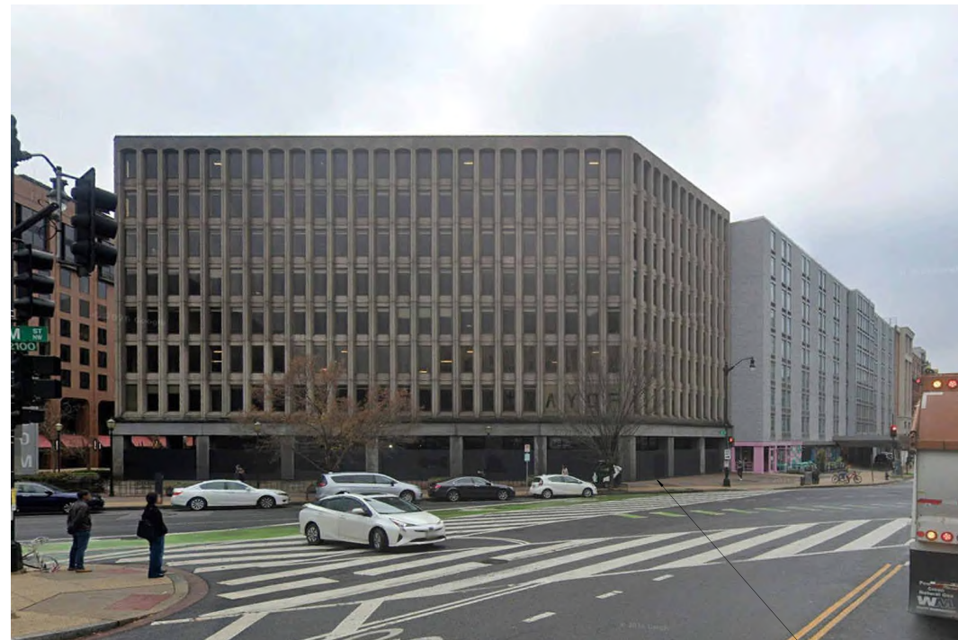
SITE PHOTO - NEW HAMPSHIRE AVE LOOKING SOUTHEAST
