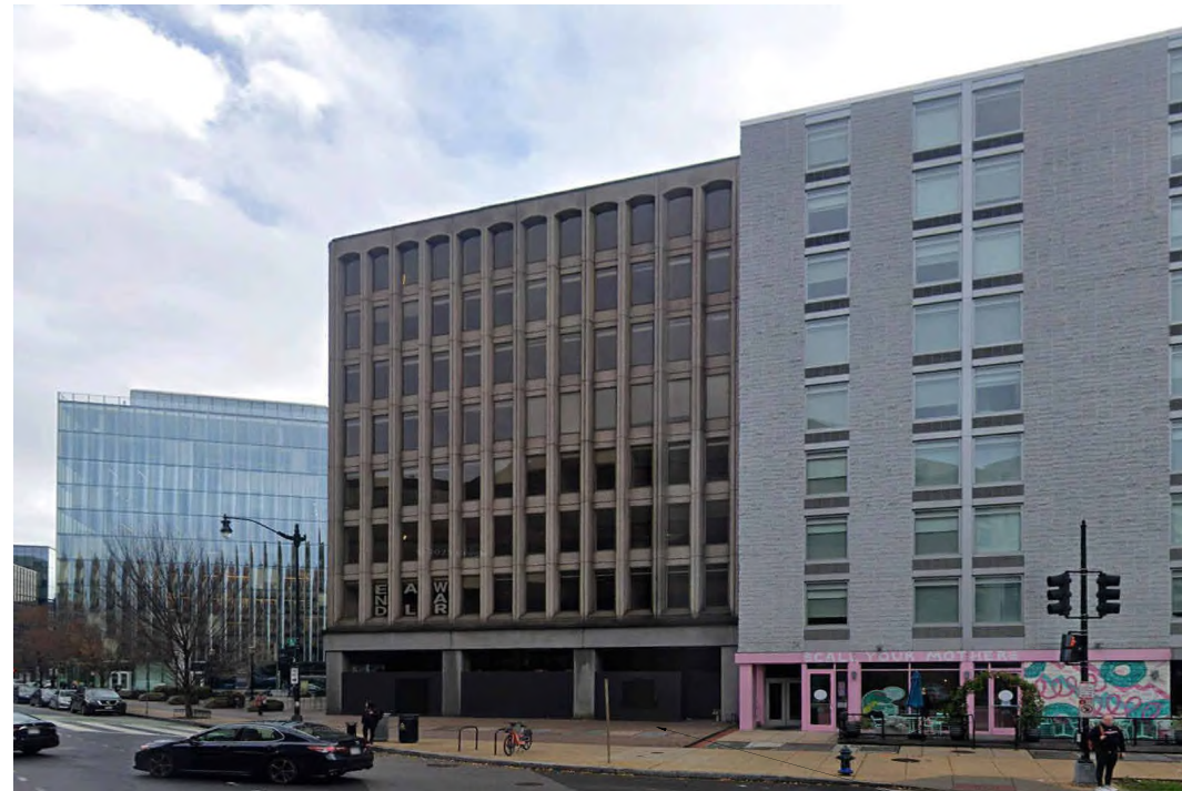
SITE PHOTO - M ST LOOKING EAST
